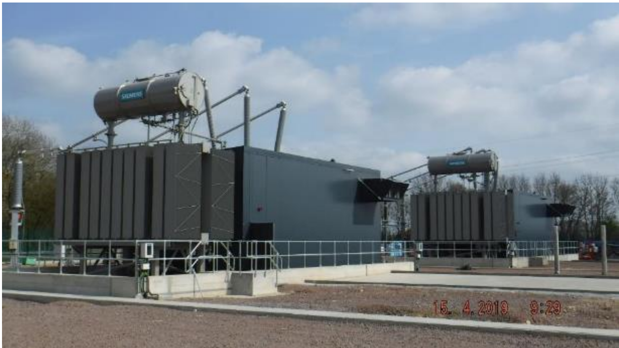
Plate 6.25 Example of Shunt Reactor Building to House Reactive Compensation Equipment (example taken from East Anglia ONE substation)
