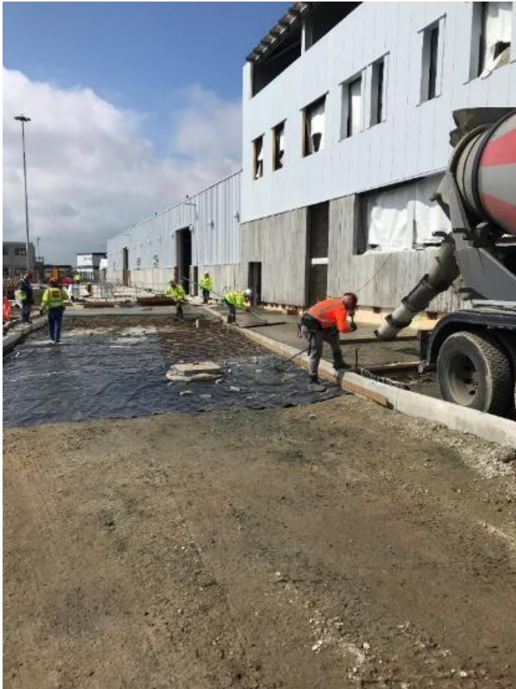
Plate 6.28 Construction of Substation Operational Access Road (example taken from East Anglia ONE substation)
