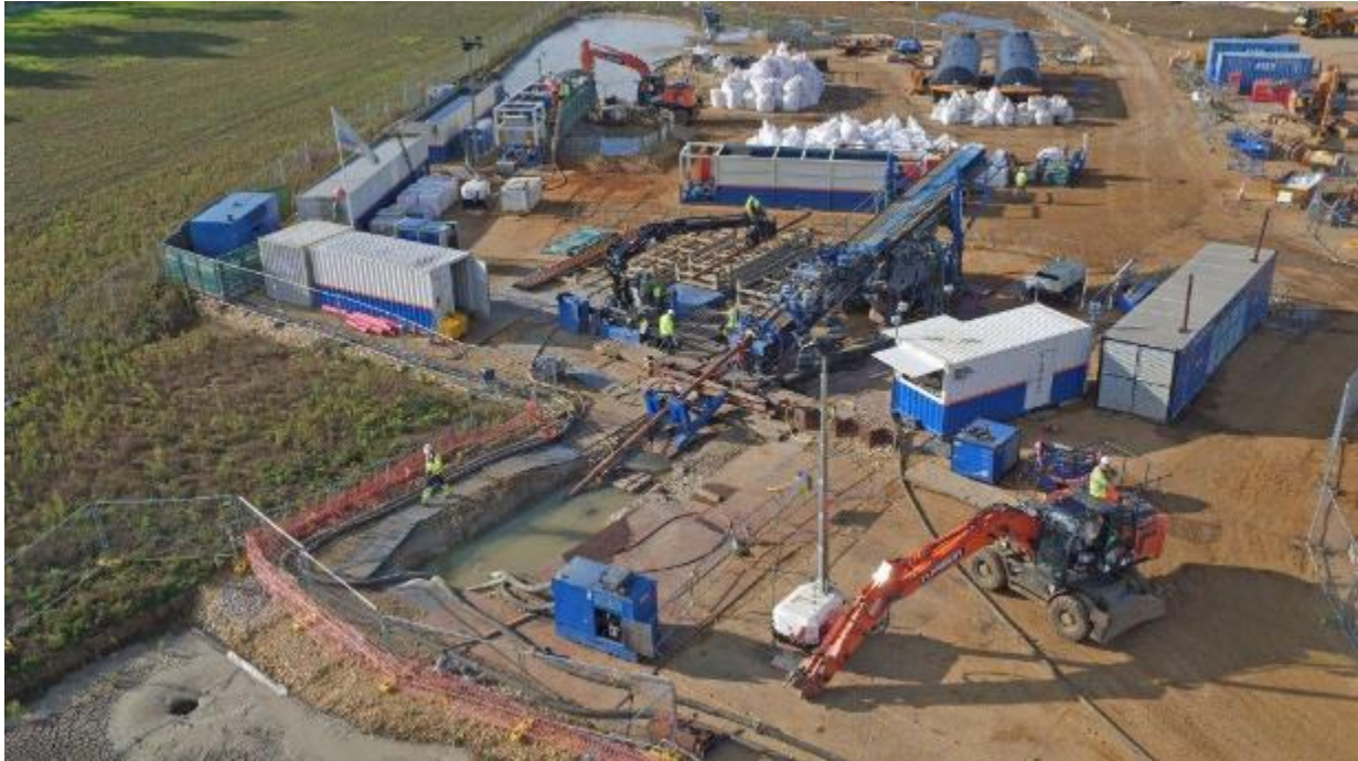
Plate 6.17 HDD landfall duct site (image taken from East Anglia ONE project)
