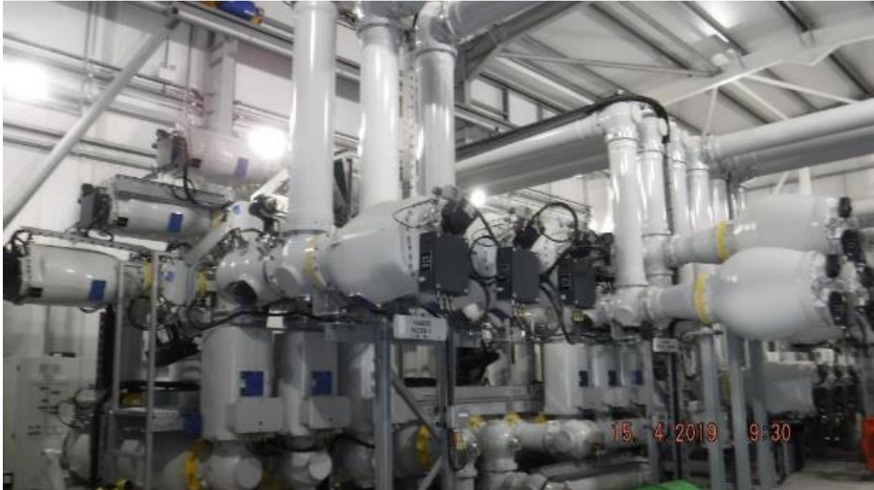
Plate 6.24 Electrical Equipment Contained within the Main GIS Building (example taken from East Anglia ONE substation)
