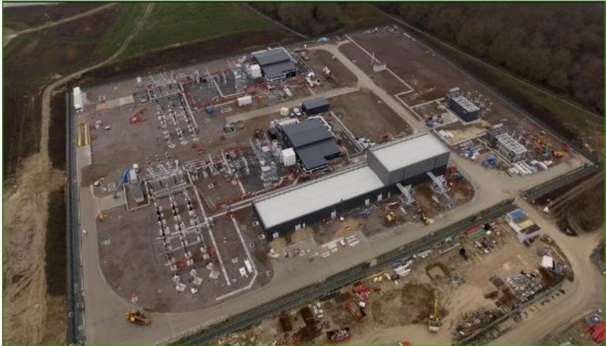
Plate 6.26 Example Layout of the Onshore Substation (example taken from construction of East Anglia ONE substation)
